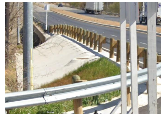
Figure 2 – MH #37342 (Viewing Northeast)
